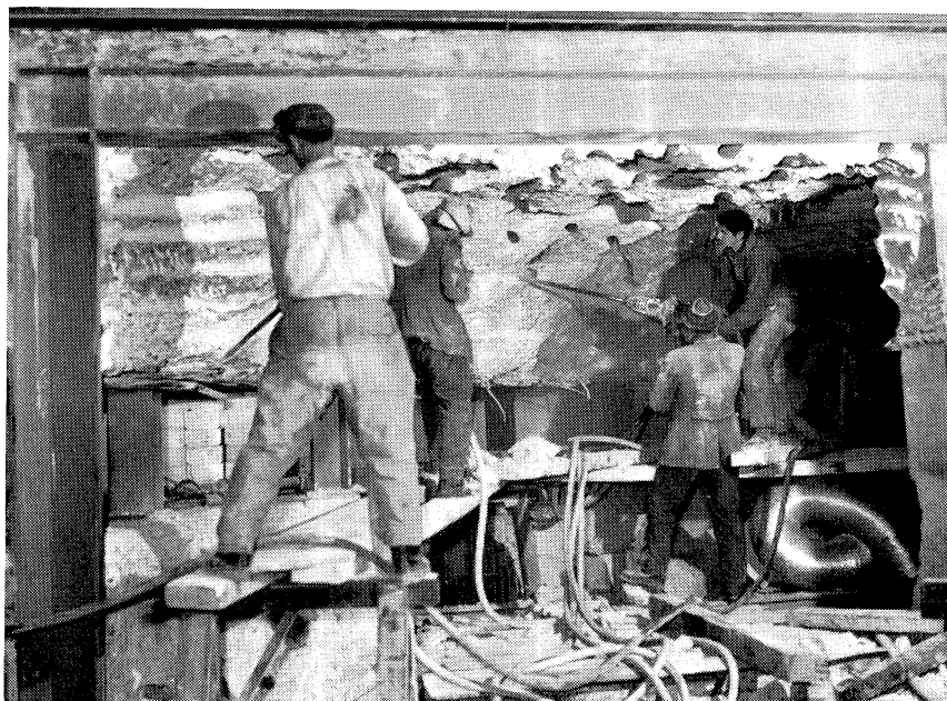
Breaking through the wall of the synchrotron tunnel was no easy task, as can be seen from this photograph. Formerly a fairly narrow horizontal slit to let through beams of particles, the aperture has now been enlarged to full height in one place to allow room for beam-transport magnets. Full shielding is ensured by movable concrete blocks, as in the other beam areas.
